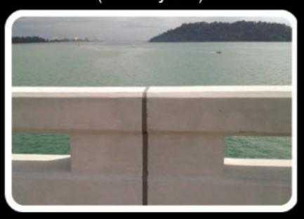
➤ Poor UV resistanceSealant cracking (PU Sealant)
